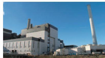
Walter Scott, Jr. Energy Center of MidAmerican Energy Company
