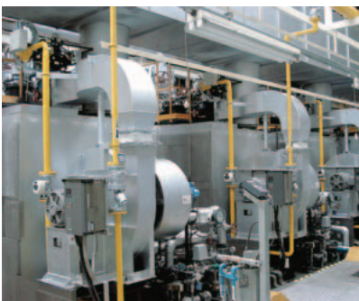
Compact natural gas-burning once-through boilers with integrated control systems
