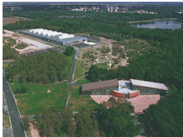
HICEF site: administration building in foreground, factory in background
