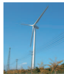
2MW downwind turbine
